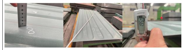
2. The sub assembly and main assembly continued today, checked the dimension complied with drawing, the diagonals were within 4mm.
